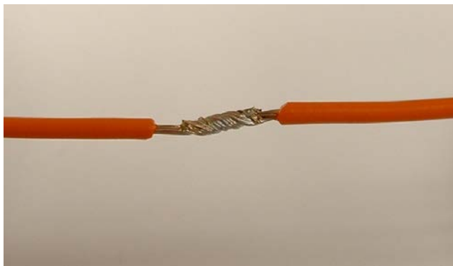
Tightly twist the two wire neatly together
