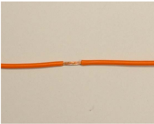
Strip a 1/2" – 3/4" section of the main wire
